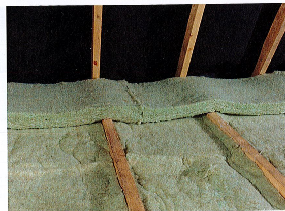
Roof insulation in a house.
